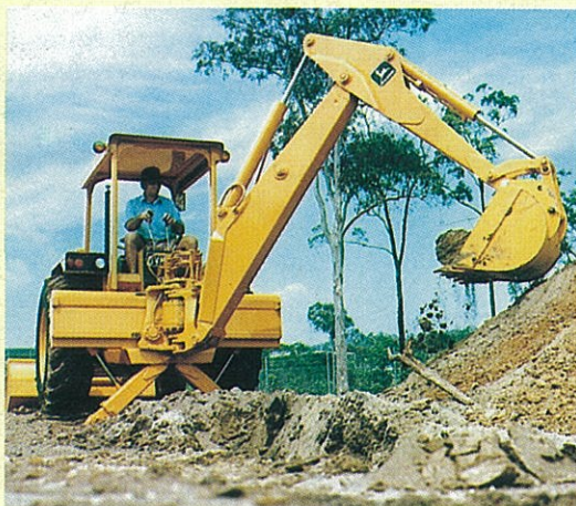
John Deere backhoe loaders.
