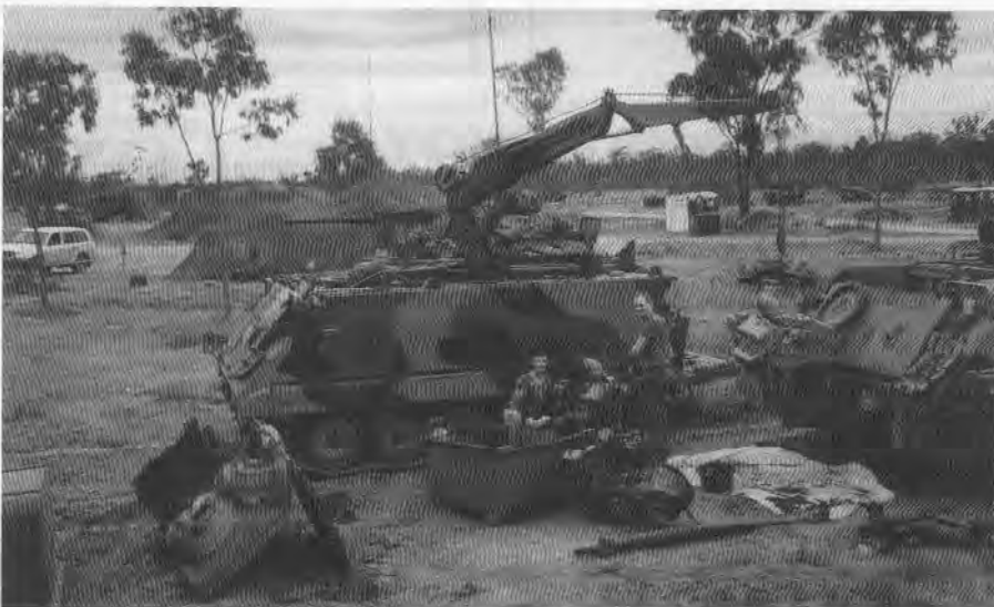
Left to right: CFN 'Thommo' Thompson, CFN Byron Kelly, CPL Tim McDougall in the middle of M113 engine change
