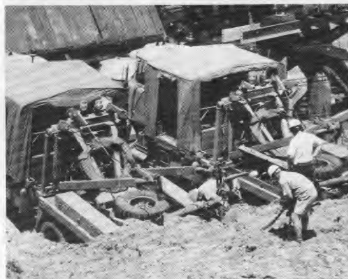
Preparing the earth bank anchor
