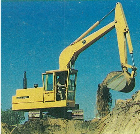
John Deere excavators.
