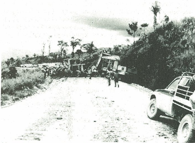
Shows SGT Dave Stewart directing the task with grader almost on the road.
