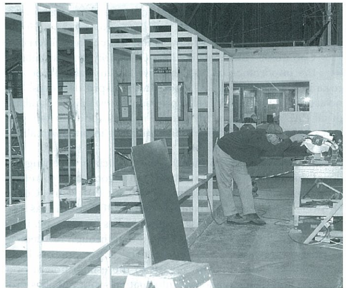
Work is under way on the new display cabinets
