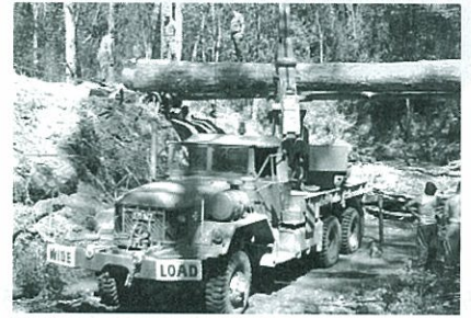
The M816 again demonstrates its versatility. Bridge building with the engineers 1980.
