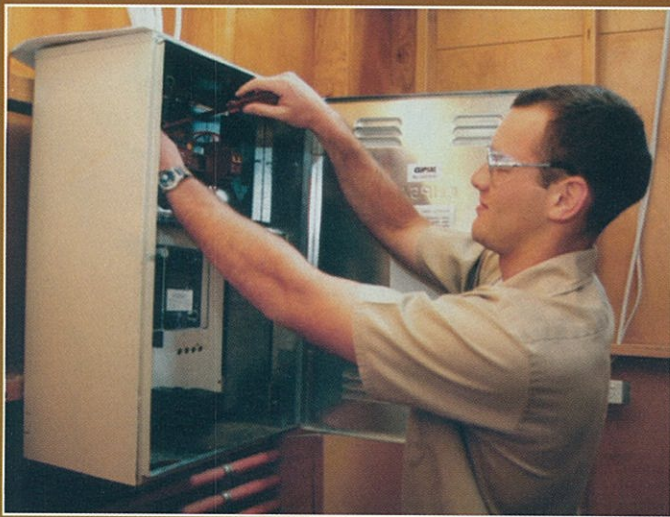
Domestic wiring training
