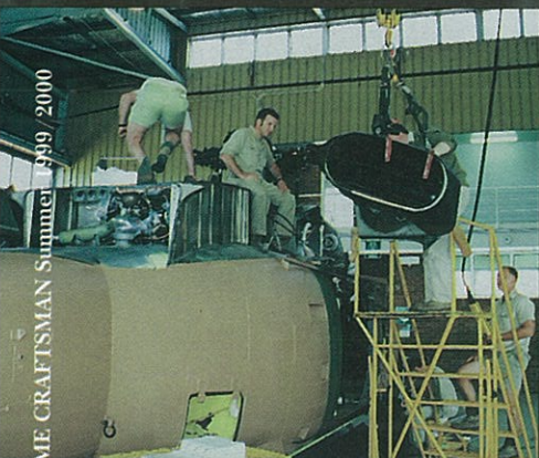
The Hover Infrared Suppressor System (HIRSS) Module being lifted into place
