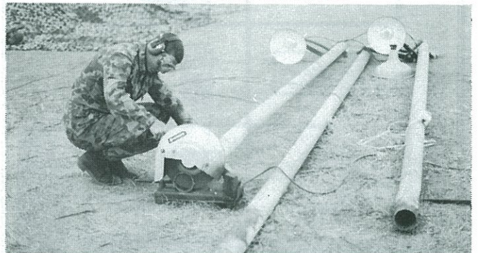
CFN Leigh Holmes (GE PL) performing repairs on racecourse light poles.
