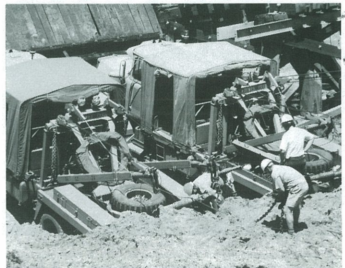
Preparing the earth bank anchor
