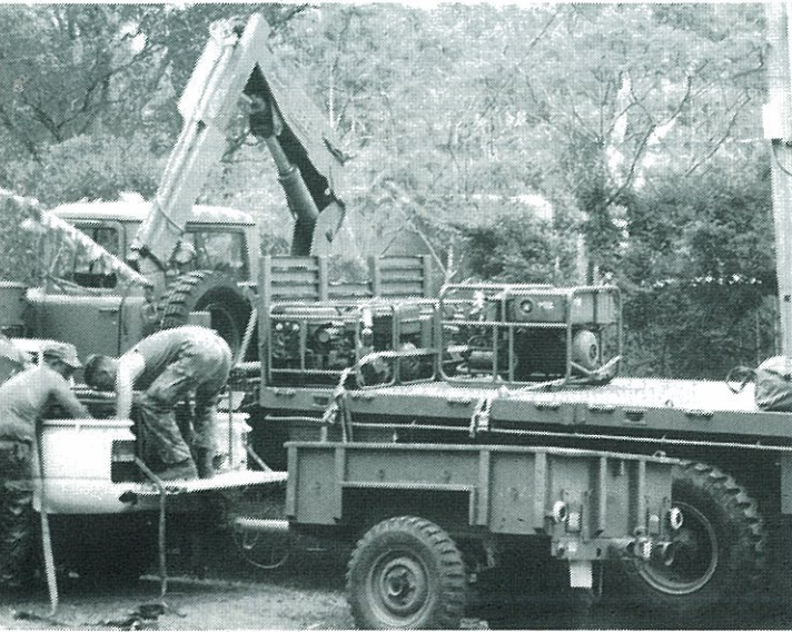
Delivering the generators by road
