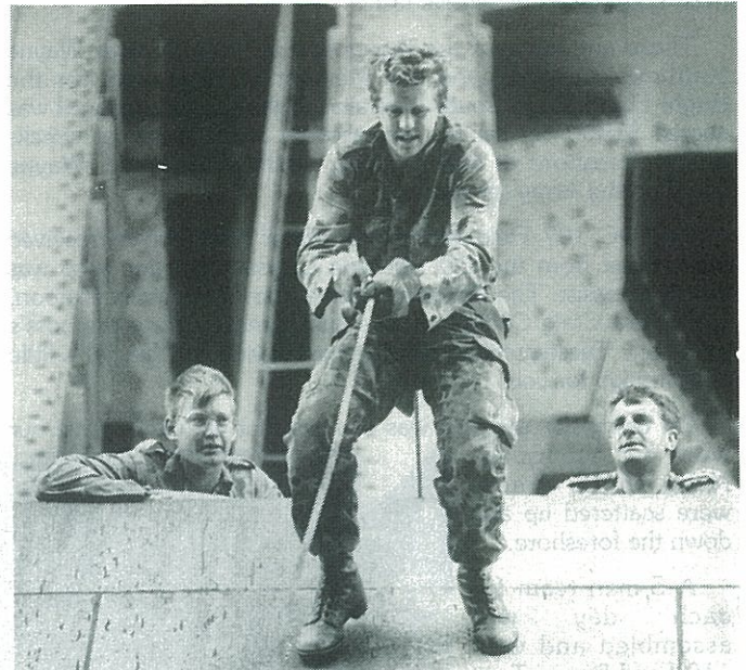
CFN Davis (left) and Capt Littame watch CFN Street Carabiner down southern pylon, Sydney Harbour Bridge.
