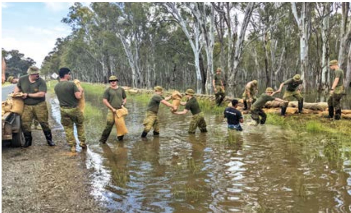
B Coy members repairing a broken sandbag levee to the north of Barmah
