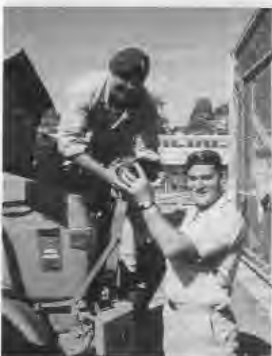
CPL Howe and LCPL Turnbull changing the alternator in a mog (no, we don't always wear our berets when working!)
