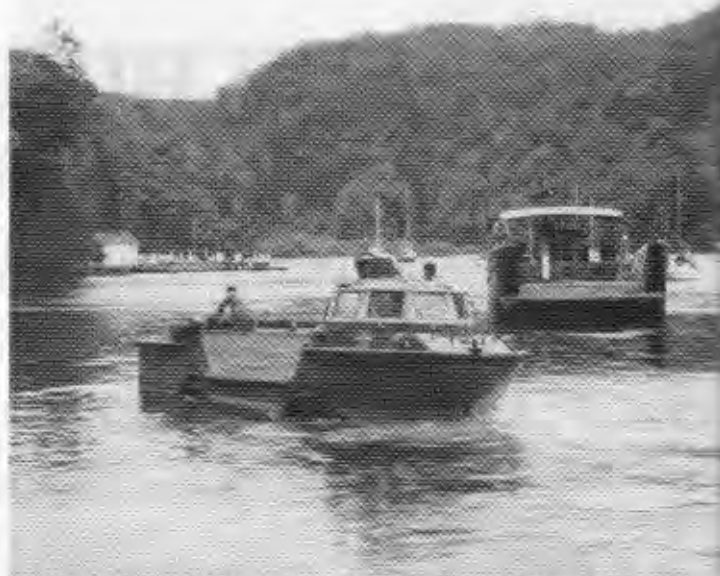
10 Tml Regt provided an LCM8 and LARC to assist in the extraction of the generators. The hills in the background were burned to the water's edge
