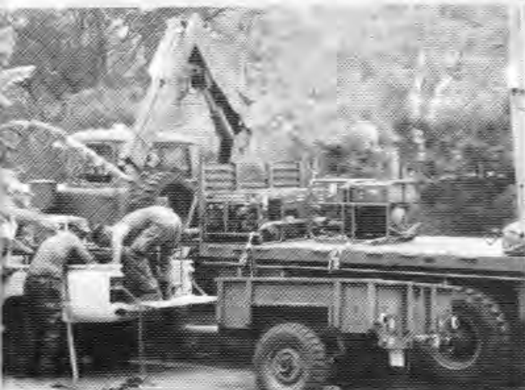
Delivering the generators by road
