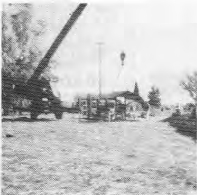
The Memorial Cairn site at the start of construction.
